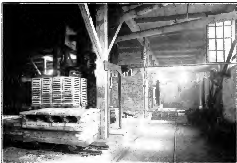
The Charge End of the Tunnel Kiln Type of Furnace. An empty and a loaded truck are seen in the left foreground
